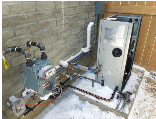
Photo B2 - Example of residential co-generation system and nameplate label
