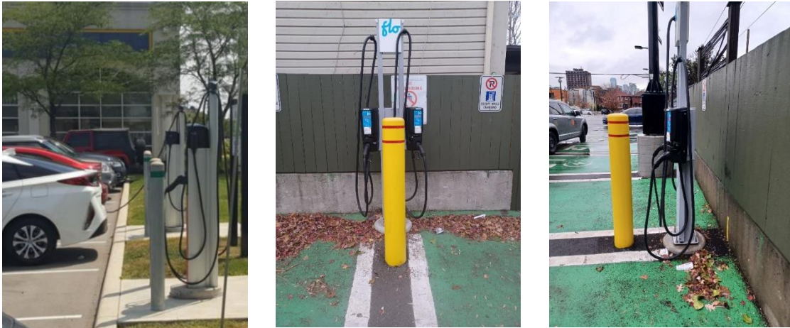
Photo B5 – EVSE protected by bollards
