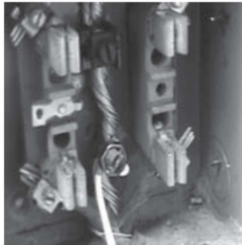
Step 2b Split-nut Installation
