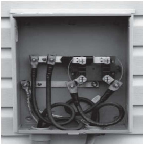
Step 2a Hi-Lug Installation
